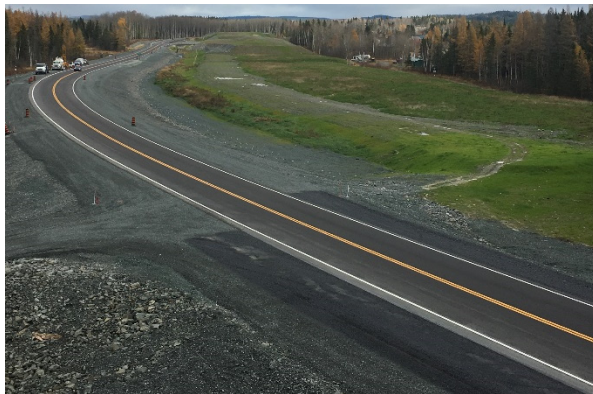
Figure 3. Photograph of the Swamp H6/H7 highway realignment, facing east
