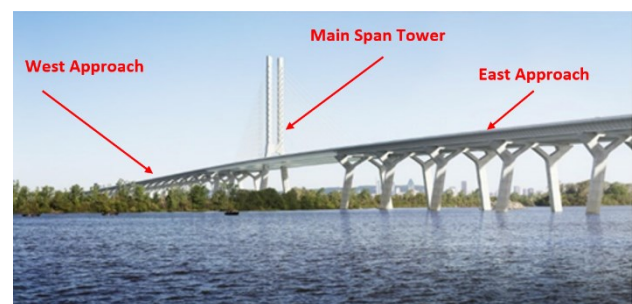
Figure 3. Main bridges segments
