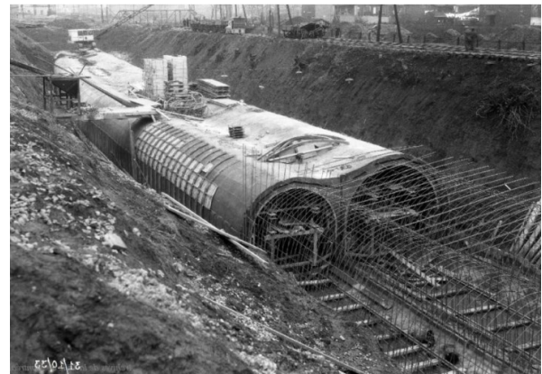
Figure 7. Construction of Collector Saint-Pierre in 1933.
