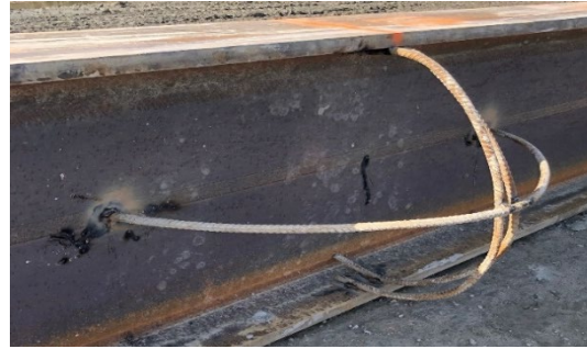
Figure 12. Centralizers on the steel beam
