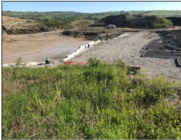
Figure 3. Drainage blanket construction on South Pond
