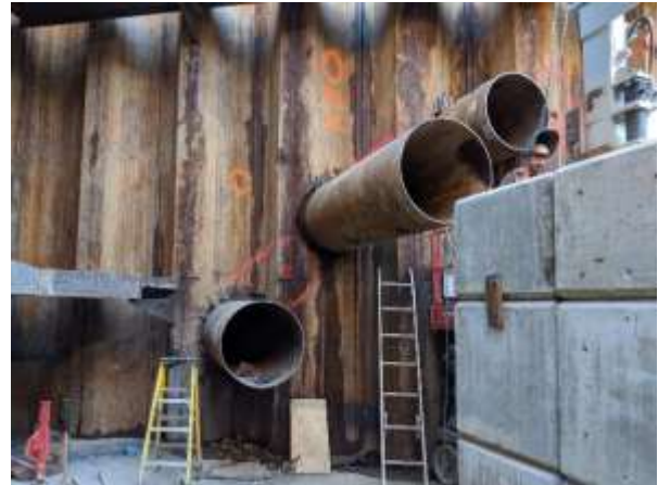
Figure 6: Installing pre-support pipes
