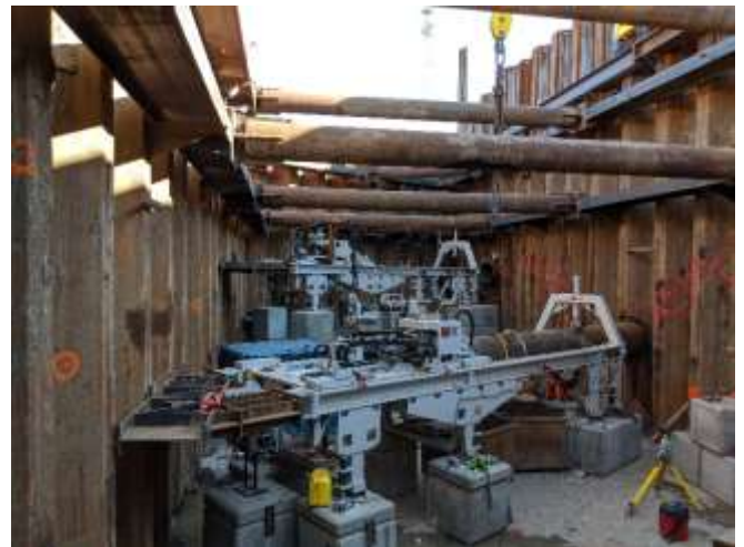
Figure 12: Shaft and auger boring machine
