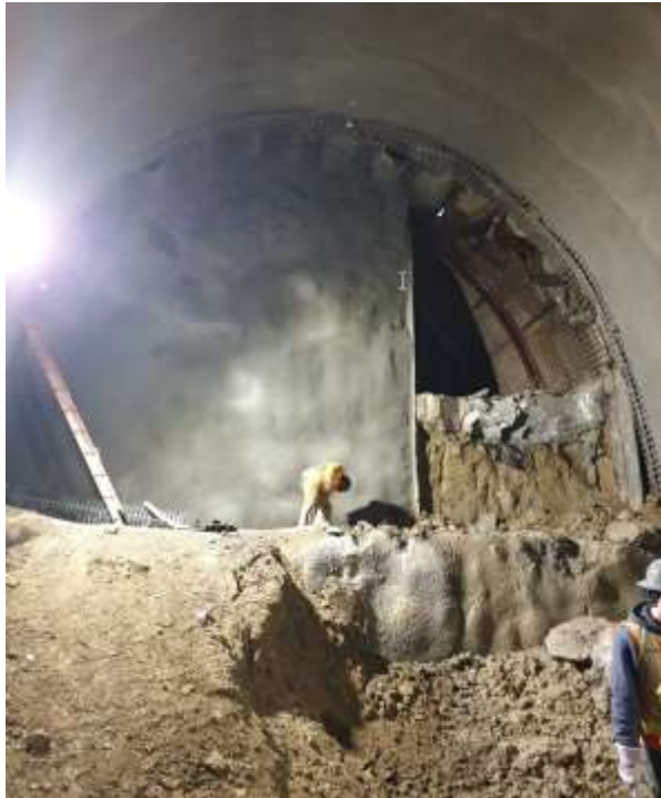
Figure 13: North tunnel break through into the shaft wall
