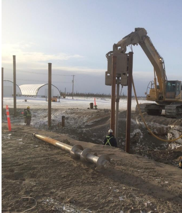
Figure 3. Helical Pile Installation with Hydraulic Wrench (courtesy of Stantec Consulting Ltd.)
