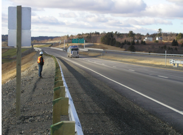
Figure 5. Completed TDA Embankment, Dec 2008
