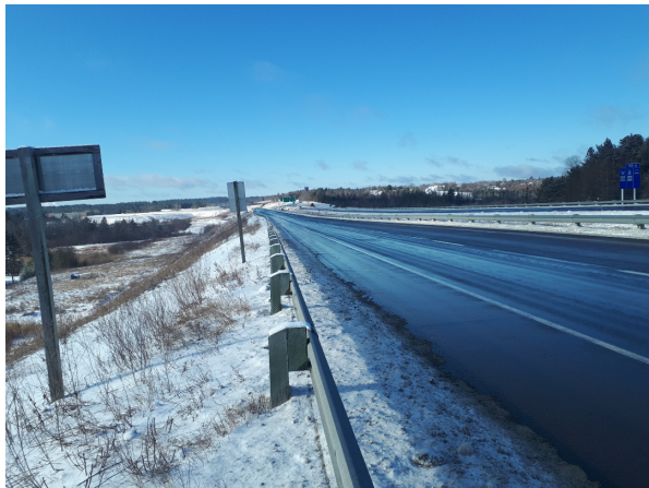
Figure 7. TDA Embankment, Jan 2020
