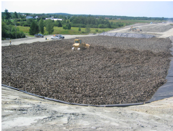
Figure 4. Placement of Bottom TDA Layer, Aug 2007
