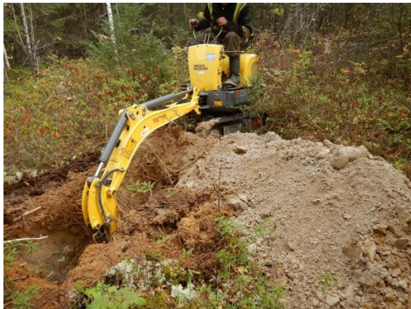
Figure 7. Mini-excavator digging a test pit into an ice-contact glaciofluvial landform.
