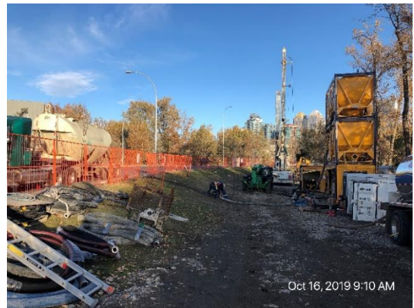
Figure 9: Site arrangement for jet grouting
