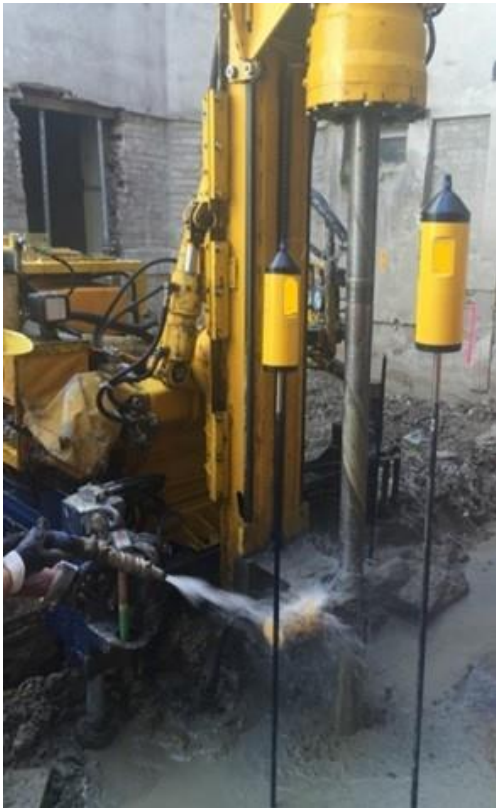
Figure 8: ACI sensors attached to embedded steel rods
