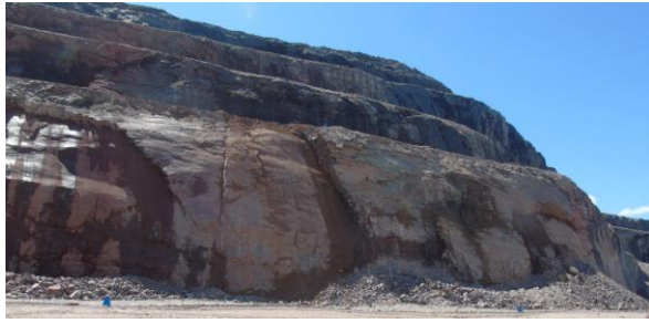
Figure 4. Slope failure and slabs observed on the southeast wall (bench 700-728)
