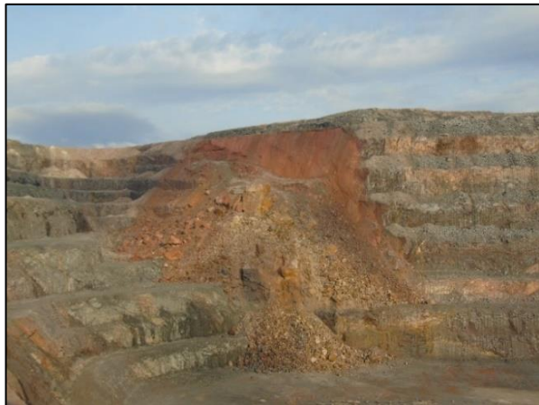
Figure 2. Southeast highwall post-failure photograph
