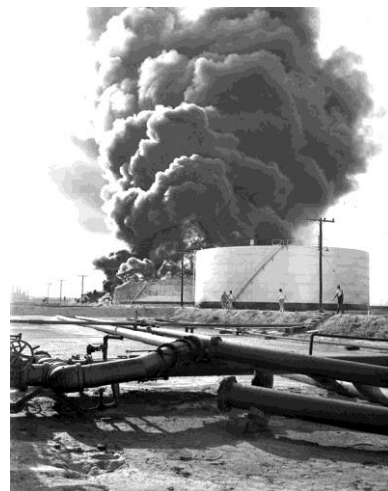
Figure 3. Explosion and major fire occurred after the failure of a fuel storage tank (API 2001)
