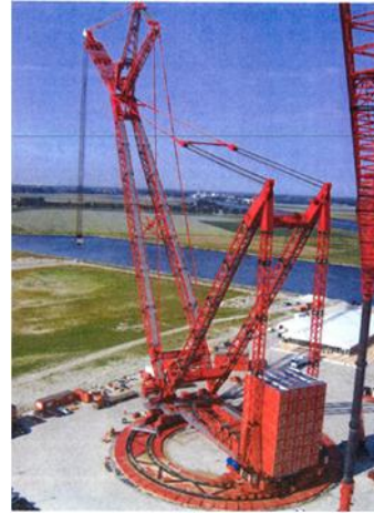
Figure 2. Photo of a PTC ringer crane
