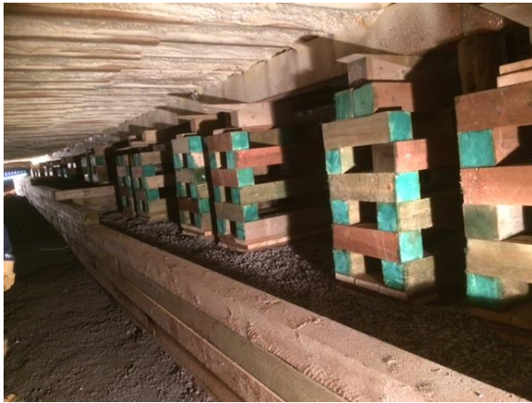
Figure 5. Wood retaining wall to hold the gravel pad
