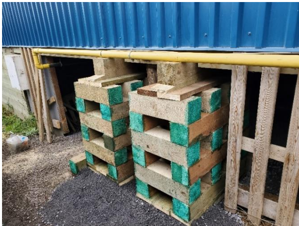
Figure 6. A typical configuration of a wood blocking
