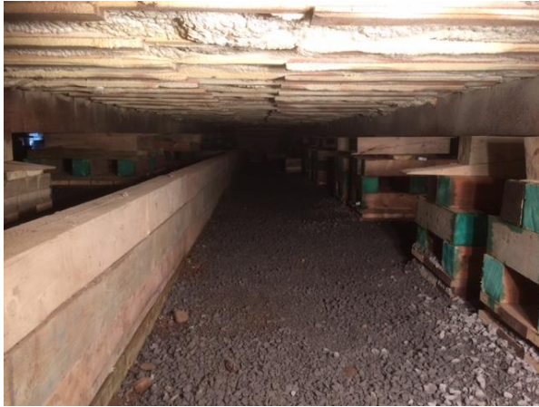
Figure 4. Gravel pad to support the wood blocking system
