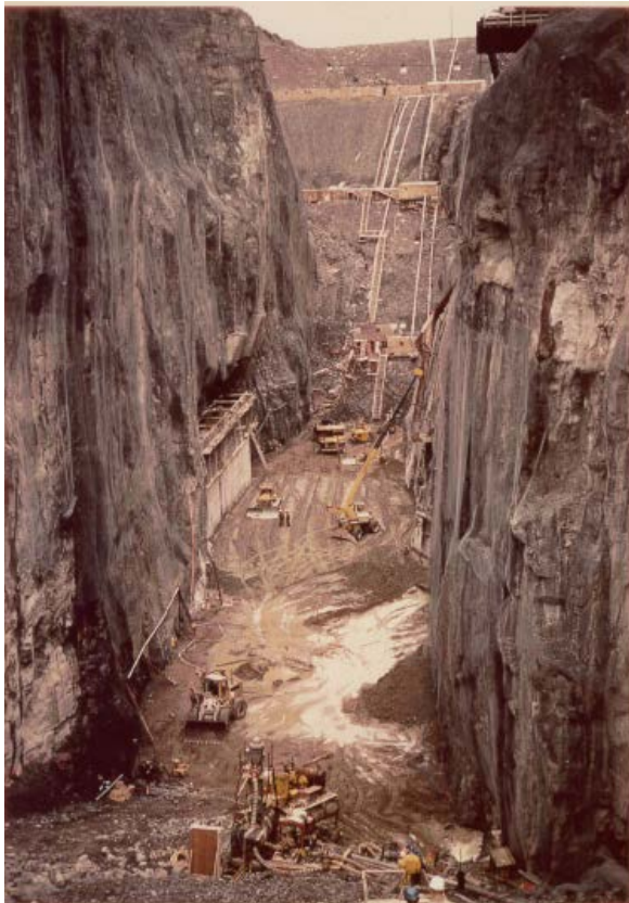
Figure 15. Lower Notch Dam, northeastern Ontario, where Casagrande, Terzaghi, Peck were consultants
