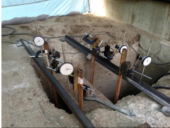
Figure 4. Pile load test set-up at Pile E-16, East Pier
