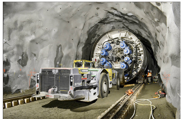
Photo 13. Tunnel boring machine ready to complete the T2 tunnel (Northern Sentinel, 2019)
