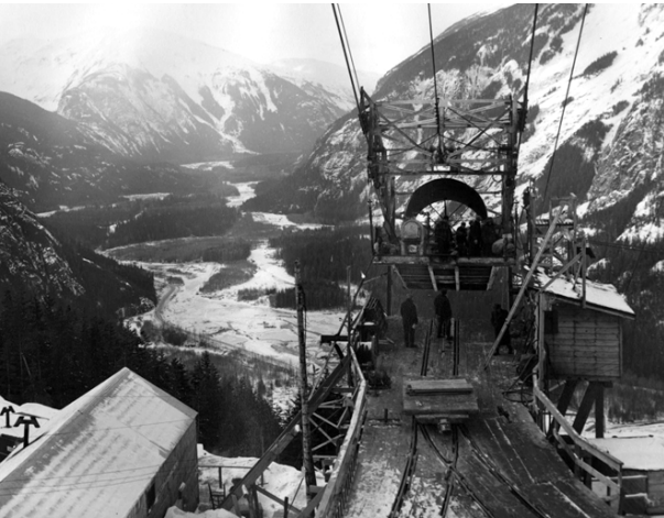
Photo 4. Tram used to get to the T1 tunnel portal and penstocks, January 1954 (Kitimat Museum & Archives)
