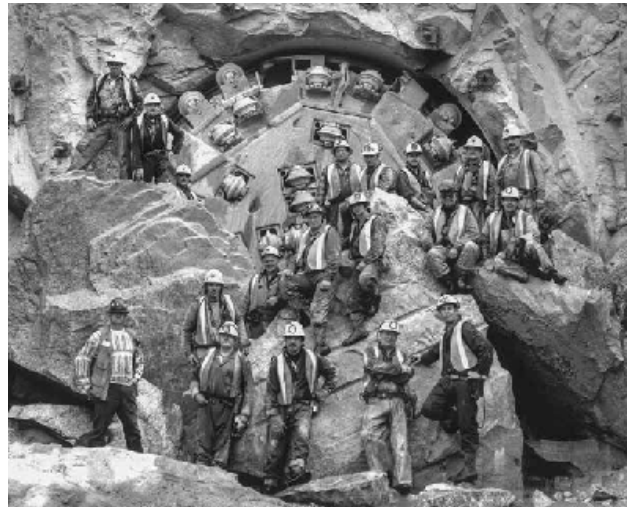
Photo 9. Partially completed T2 tunnel excavated by a tunnel boring machine (Rio Tinto)
