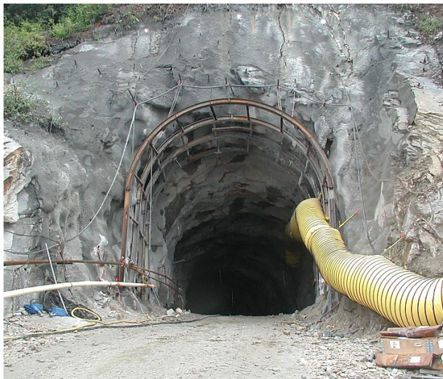
Photo 11. Access portal for T2 tunnel construction (D. Brox)
